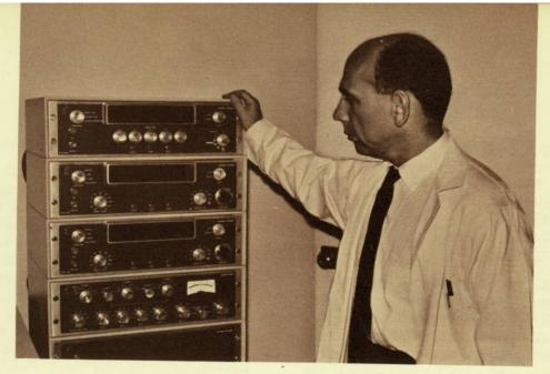
Dr. George Acs, head of the Division of Enzymology, at the console of the scintillation counter. The instrument is used to measure the radioactivity of tissue samples.
