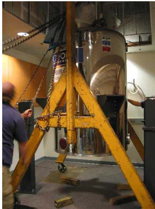
Installation of 16.45 T magnet in Hasselmo Hall.
